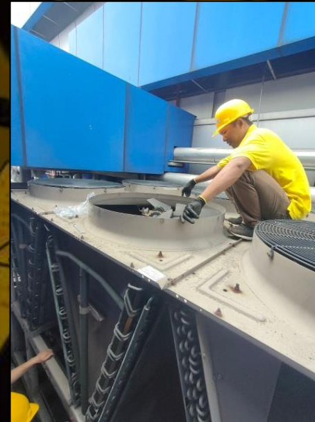
Cleaning and Repair Cooling Tower
