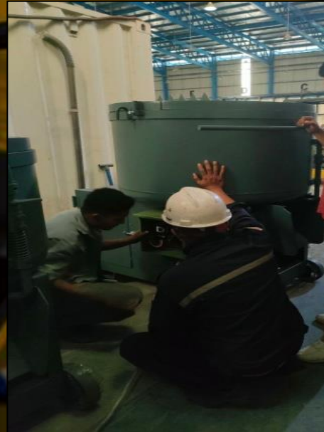
Improvement for safety and capacity up.
